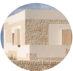
Solid limestone external wall
