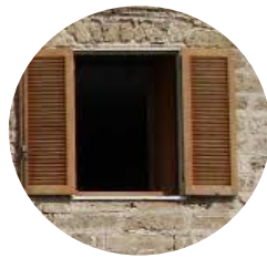
Wooden framing members
